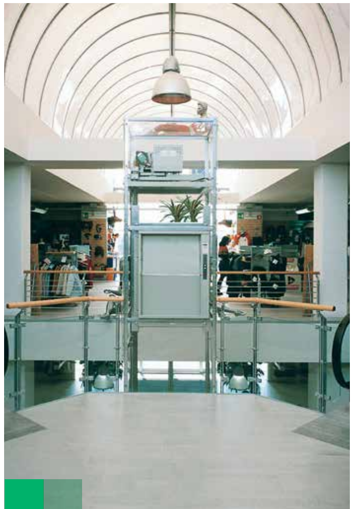
Installation in a clothing shop (Italy), model 50 kg, glass cladding and standard car in RAL 7038.
