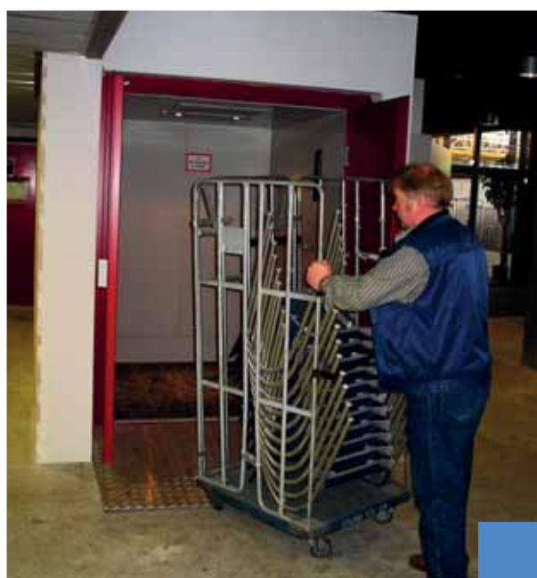
Installation in a sports centre (The Netherlands), model 1000 kg, special red coloured finish (different colours available).
